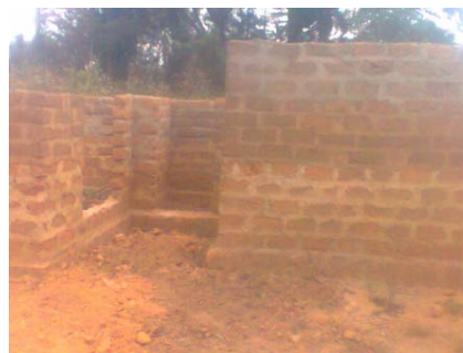
Figure 2: YAEHD Agri- Processing Center's processing facility under constructed in Montserrado.
