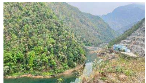
Chiang Muon hydropower plant, Muong La district: Photo credit: Trang Chu
