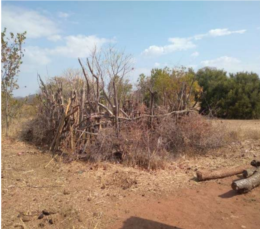
Figure 18. A poorly constructed and weak livestock kraal in Nyaminyami ward 3. Photo: [REDACTED]
